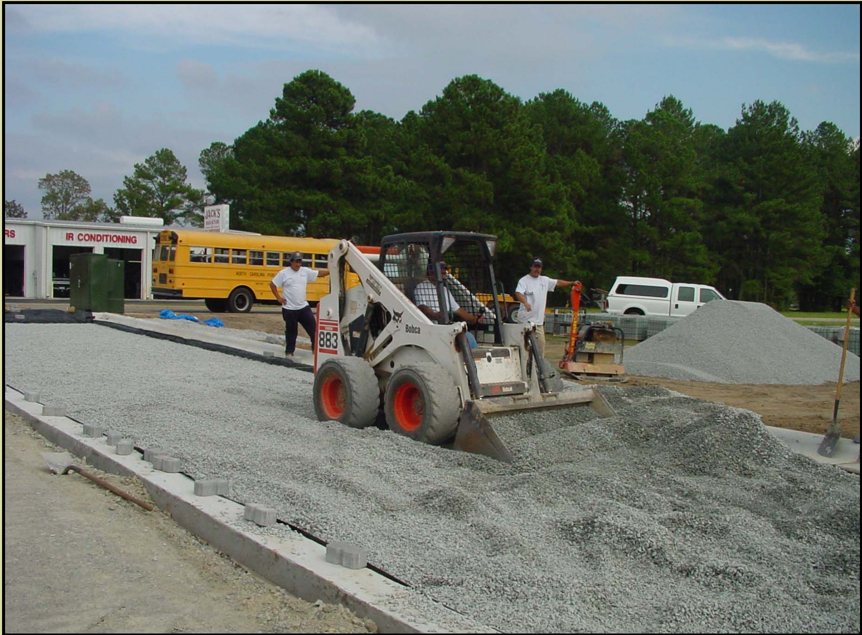
Final grading of base material
