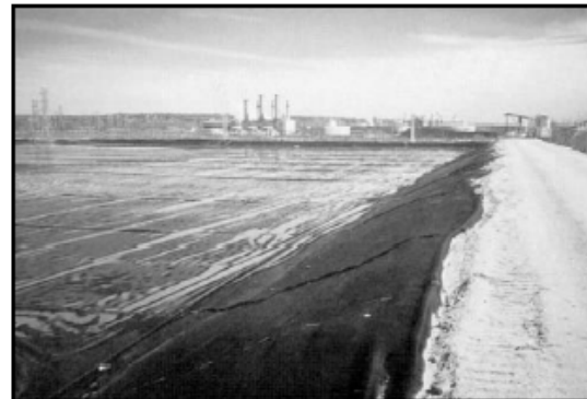
Geolon® HP-Series Geotextile used in pond closure application
