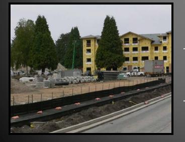
Erosion and sediment control.
